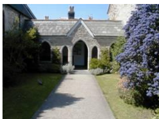
Porch entrance of St Peter's
