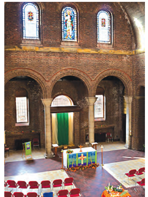
Windows restored at St Cuthbert, Copnor
